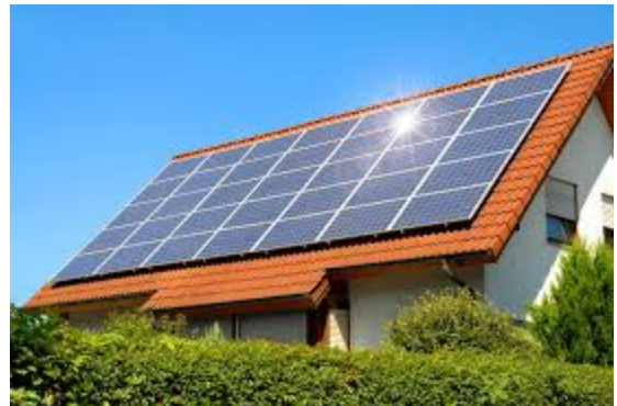
A solar power roof (Source file photo)
